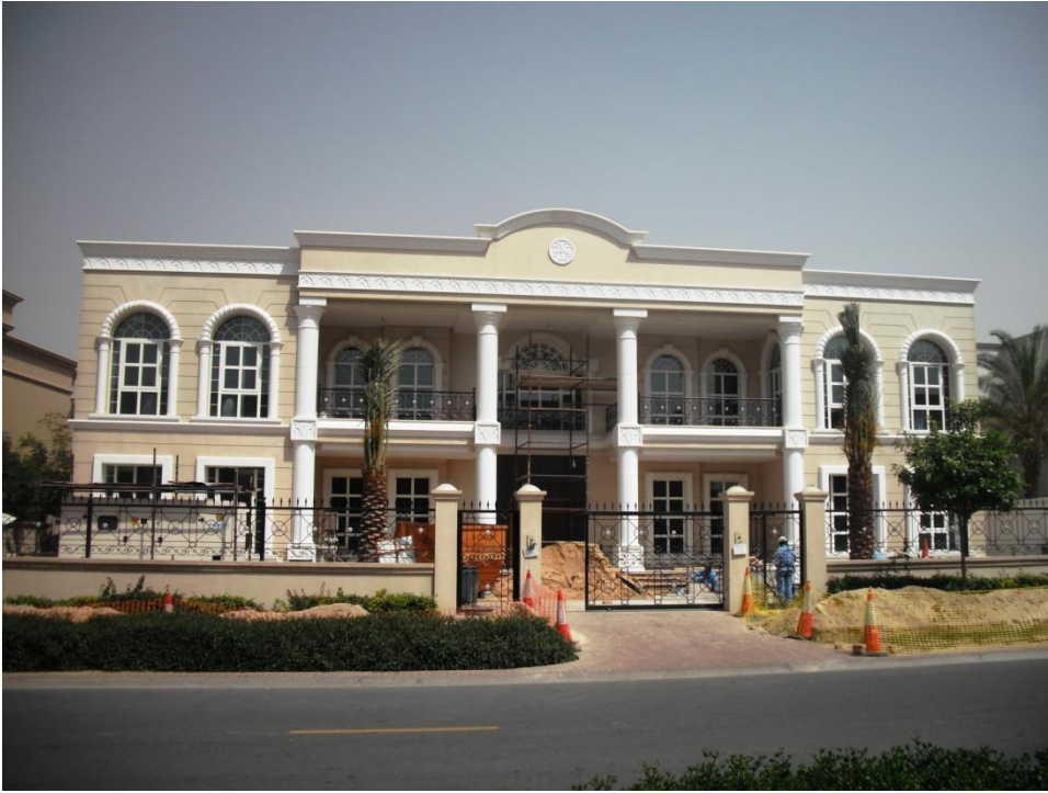
Decorative GRC Works for luxury Villa Emirate Hills (HT24) Dubai.
