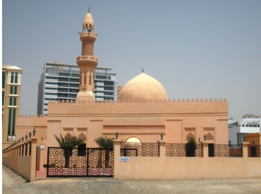
Decorative GRC Works for Mosque at Al Barsha Dubai
