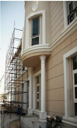
“GRC Works with Steel Structure” For Landscaping
